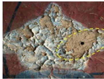
(b) A wet-dry cycle leads to the peeling of mural paintings [56]
